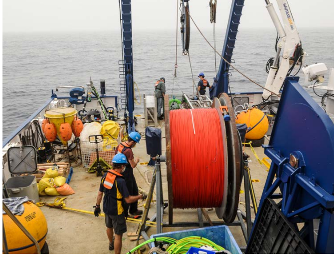
FIGURE 4 (left). Deploying cable to connect tsunami array at Cascadia Basin. Image credit: ONC
