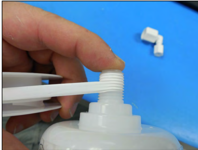
Figure E-74: Wrap Threads with \frac{1}{4} " Teflon Tape
