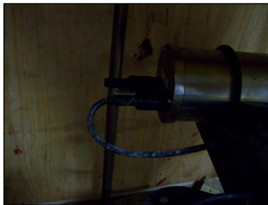
Figure 6.1-1: Results of Poor Rinsing After Deployment
