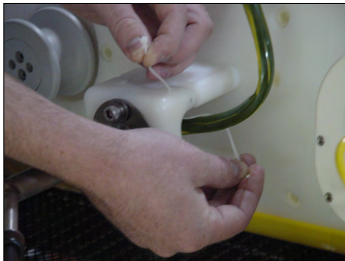
Figure 4-17: Secure Excess Cable
